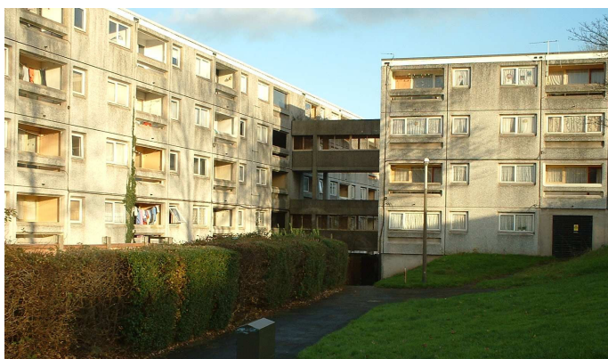
Photo 1 – Example of deck-access flats
